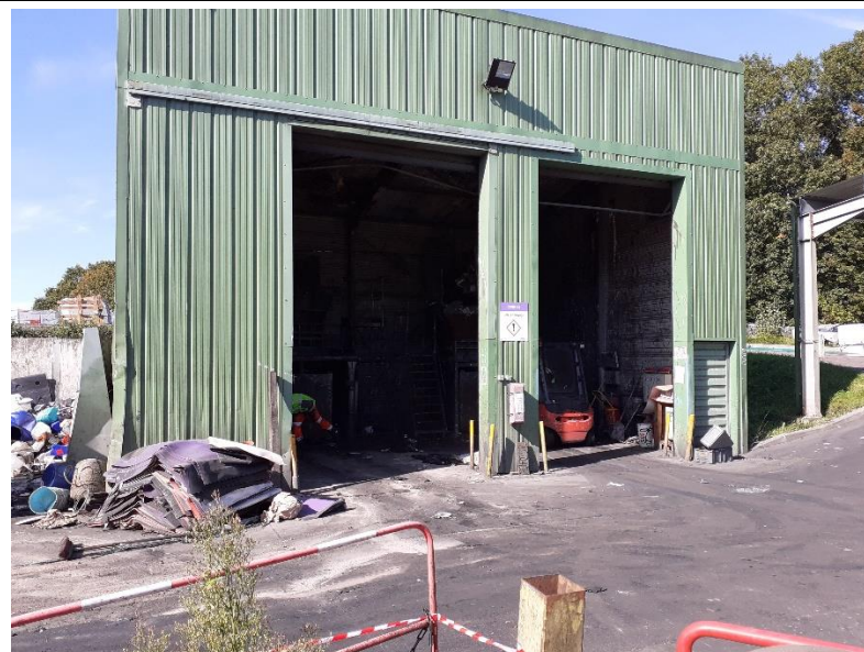
Photo 10 : Zone Z10 - Broyage
